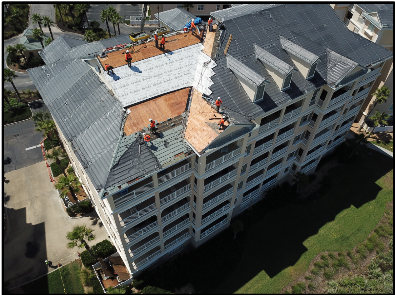
Figure 7. Photograph showing multiple roofers reconstructing a roof.
