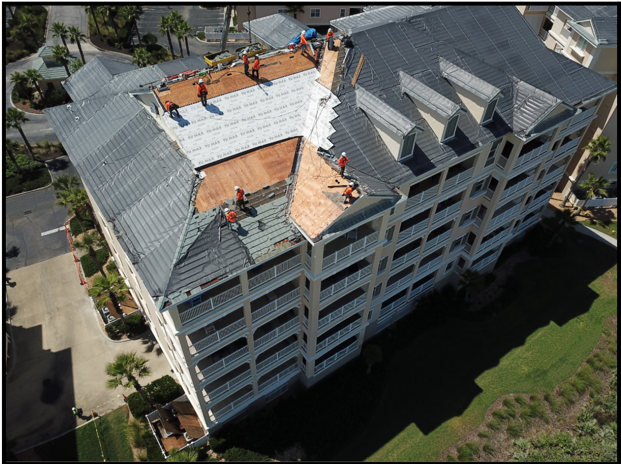
Figure 7. Photograph showing multiple roofers reconstructing a roof.
