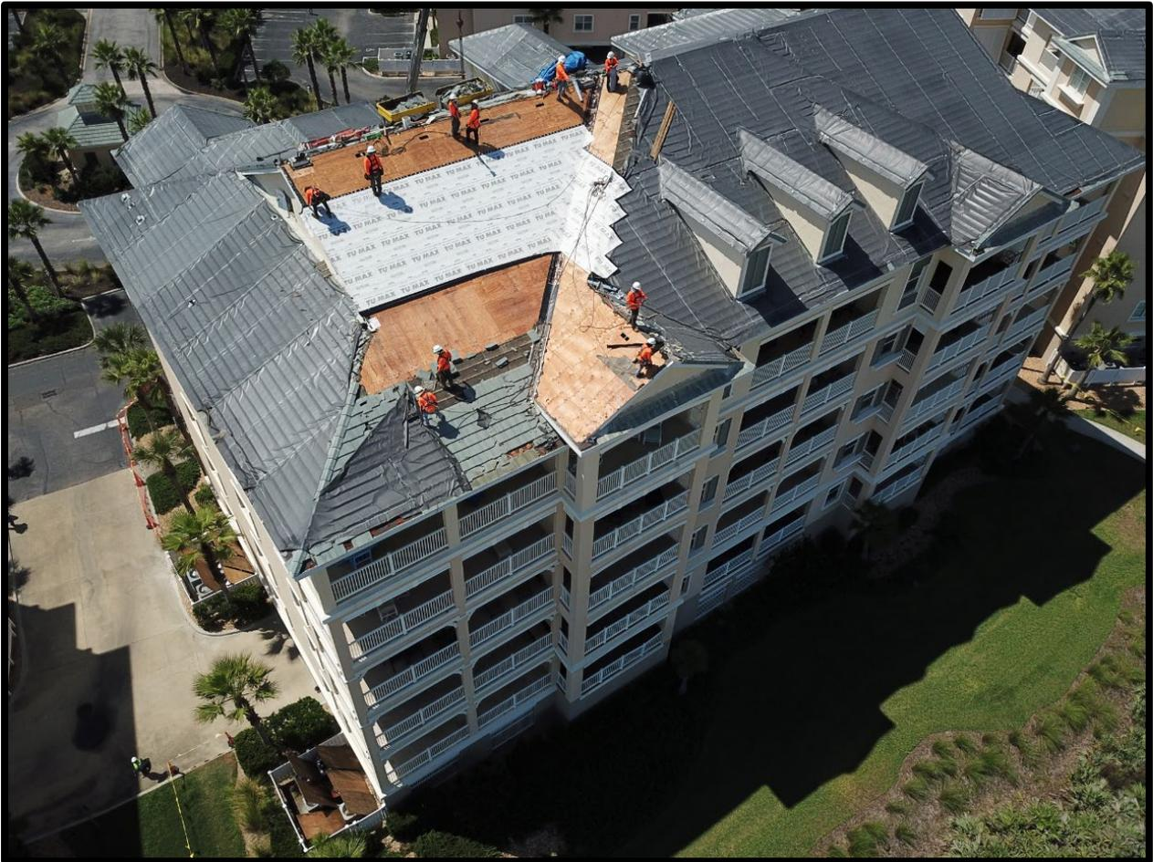
*Figure 7. Photograph showing multiple roofers reconstructing a roof.*
